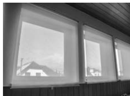
Detail oken po instalaci rolet
